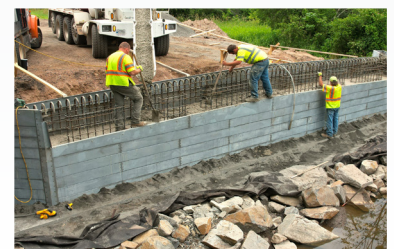
Ready-mix concrete placed in abutment.
